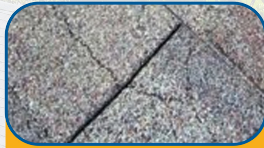
Cracked Shingles
