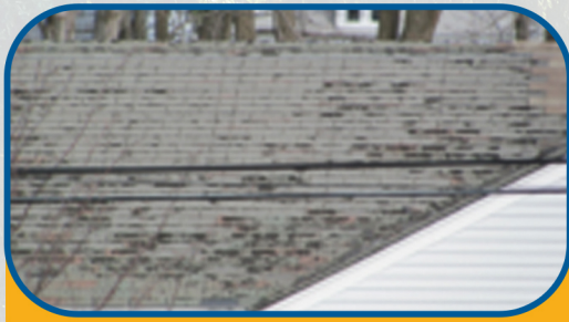
Roof is over 15 years
